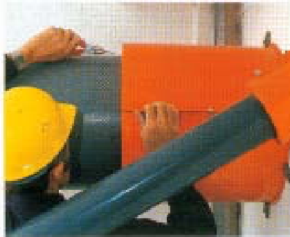
KBS Pipe Seal M installed on 500mm diameter pipe
