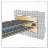
Transfer measurements onto mineral wool panel, but add about 3 mm on height and width of panel (this will result in a tighter fit). Now cut panel into as many pieces as necessary to fit in between the wall opening and cable trays as well as between cable trays.
