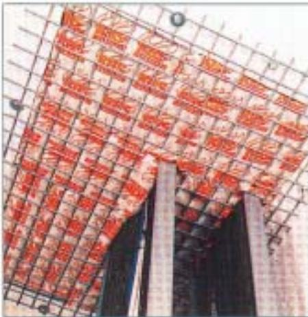
Place KBS Sealbags lengthwise and flat onto the wire mesh, layer after layer. This allows any tight spaces to be filled.
